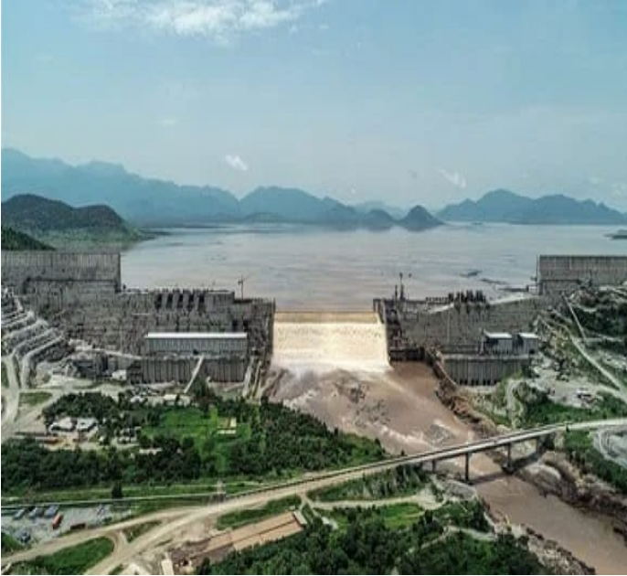
The Dam under Construction on Laga Abbayyaa (River Nile)
